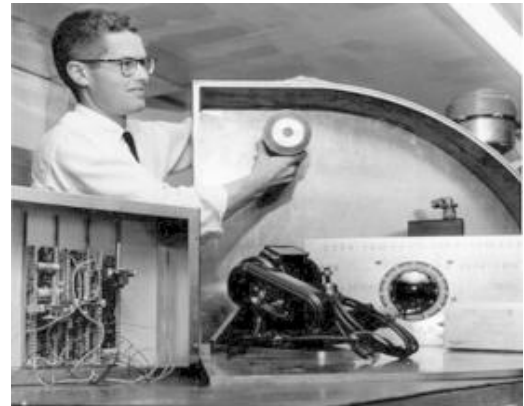
Sid Nebeker building the first high-speed rotating mirror camera for the Cordin Scientific Imaging Company, 1959.
